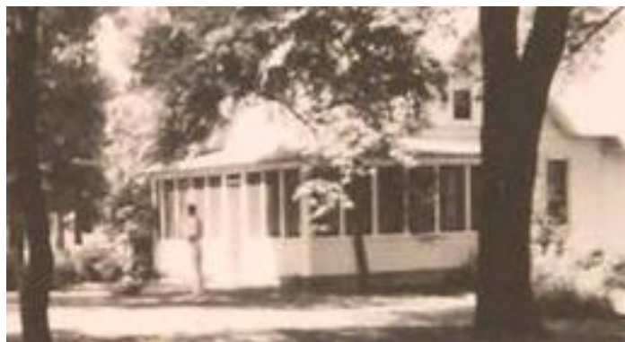
Pictured here is the former Lundberg farm house which was home to several generations of the family from 1906 up until 1978.
