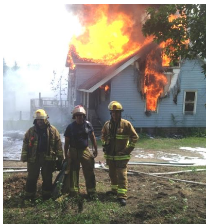
Firemen stand by the home, once owned by Carl Holmberg, being razed in a controlled burn. Photo by Josh Wing, new owner of the land.
